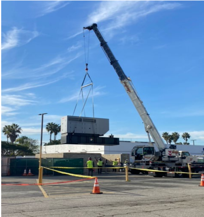
Campus Police Generator Installation
