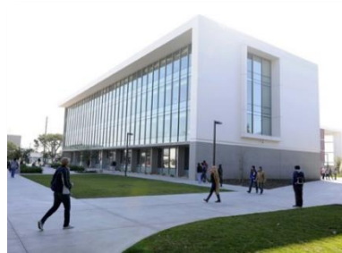
Math Business Allied Health ("MBA") Building
