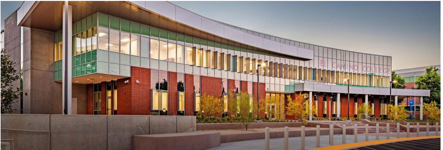
Entrance - Administration Building
