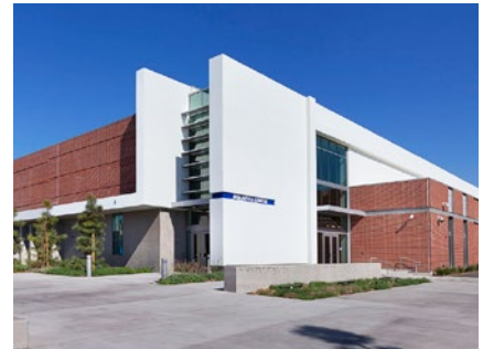
POOL/CLASSROOM COMPLEX Completed: February 2021 Cost: $50 million
